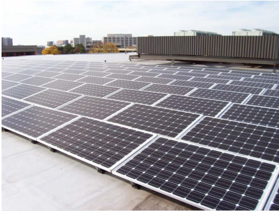
Continental Electrical Construction Company installed a 55kW solar photovoltaic system on the roof of their facility in March 2015.
